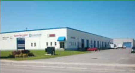
East Ottawa - Warehouse
