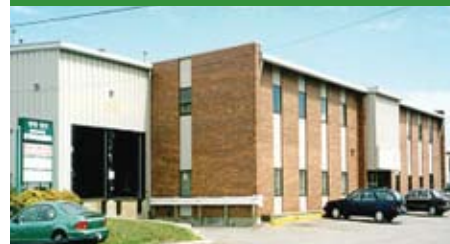
East Ottawa - Warehouse
