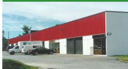
East Ottawa - Warehouse
