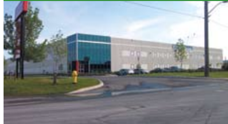
East Ottawa - Warehouse
